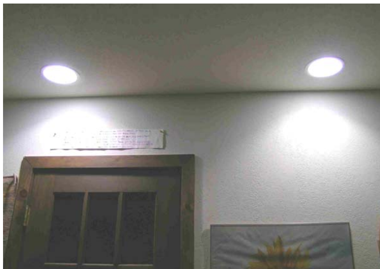
Figure 14. Light distribution with white reflectors and CFLs
