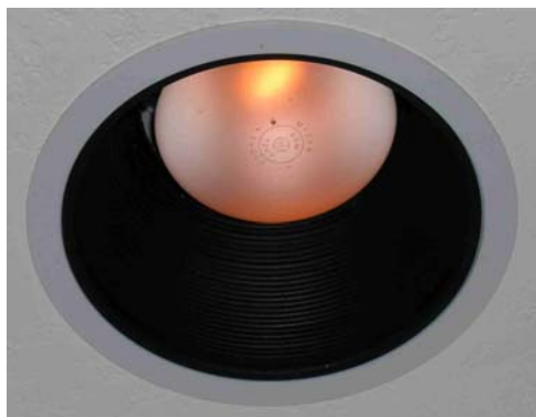
Figure 12. Black reflector with incandescent flood lamp
