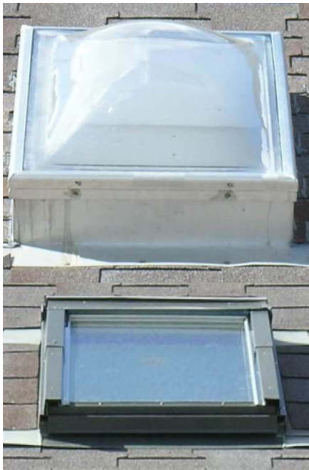
Figure 20. A fixed skylight with a double wall plastic dome is shown at top and a double-glazed skylight that may be opened to provide ventilation is shown below.
